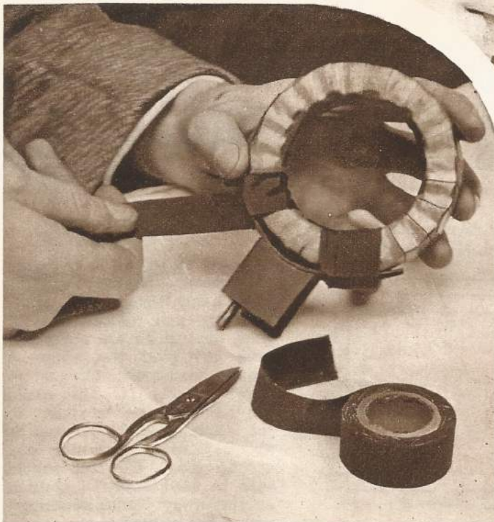
Figs. 9 and 10.—This is a good method of attachment (covered by Burndept patents) employing a binding of adhesive tape and a segment of fibre.
